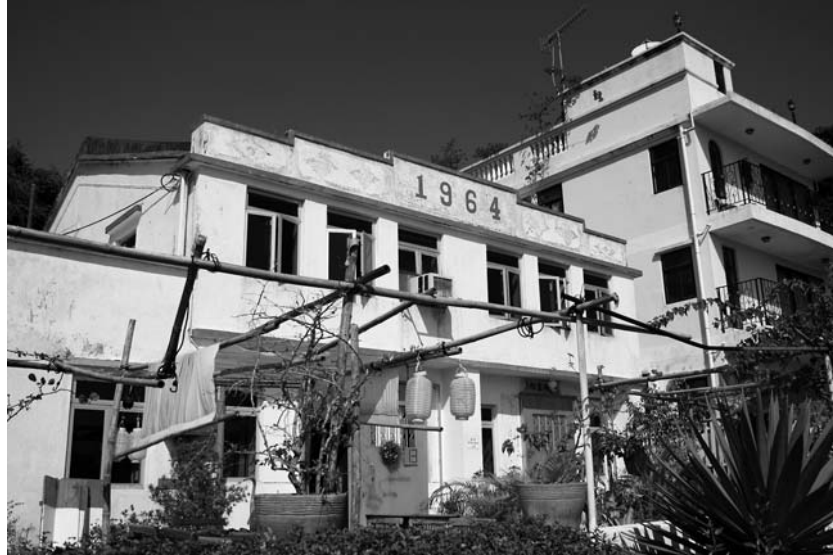
Figure 4.1. Three-storey 'village houses' in the New Territories. (Photo: Shu-Mei Huang)
